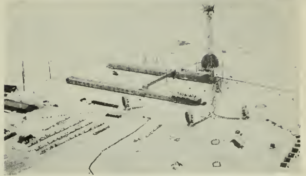
THEY DEW IT—Aerial photo shows USAF manned Dew Line station that is part of our northern defense.
